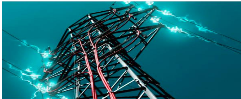
Figure 1.2 Electricity transmission line
